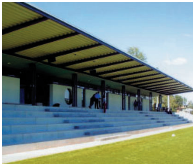
The first smaller stadium by the prefabricated construction method: Hertha BCS Berlin is building it on the throwers' training ground close to the Olympic Stadium for the club's young talent teams. For building the changing rooms integrated into the spectator stand, the Berlin branch of Otto Quast Fertighbau Sachsen utilised the monolithic wall system "Poraform".
